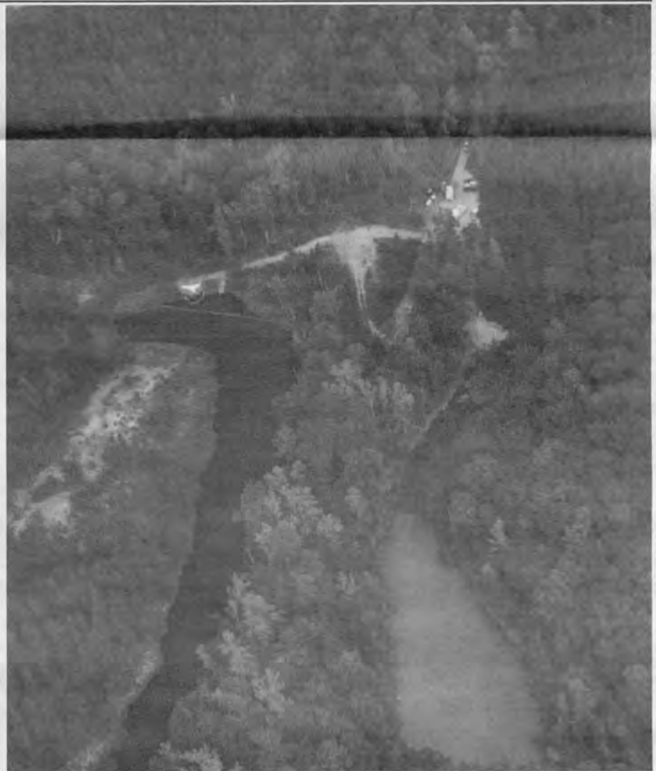
Mining retention ponds near the site of a leak in Colonial Pipeline's Line 1 Photo Credit, Colonial Pipeline
